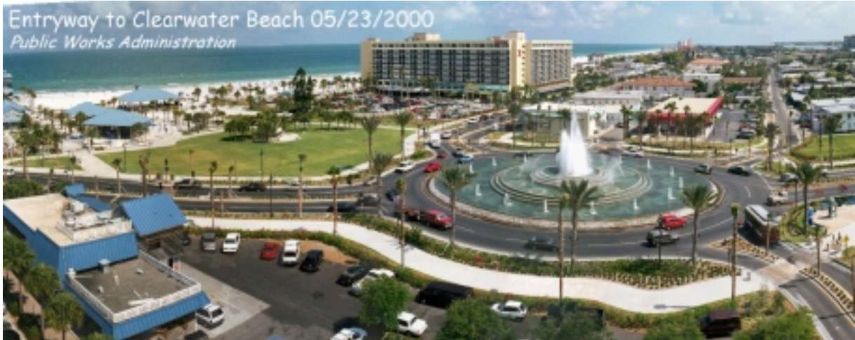
This shows the Clearwater Beach Entryway Roundabout and surrounding area (Photo by Ken Sides)
